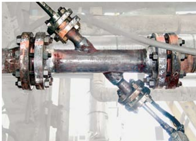
FIG. 2 Ultrasonic flowmeter body in delayed coker furnace feed line.
